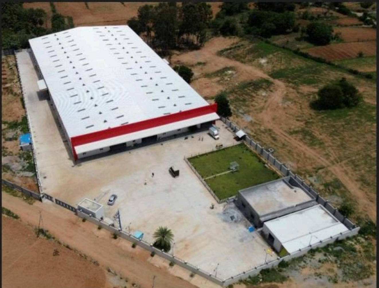
Overall View real time in Site
